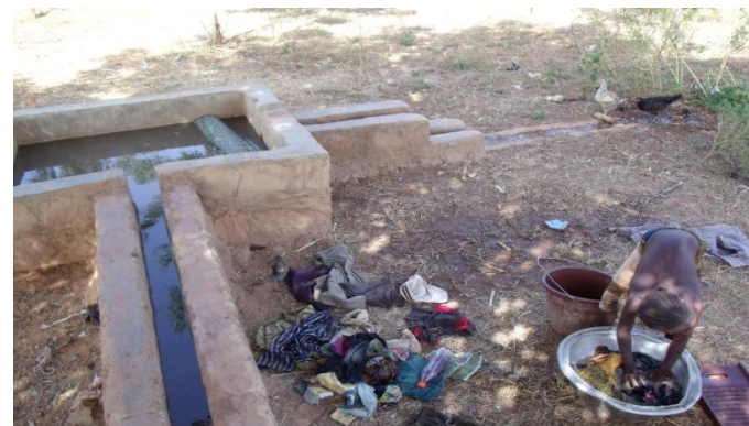
The existing washing facilities
